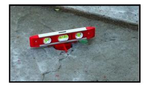
Level the Base inside the hole with a carpenter's level in two directions 90 degrees apart. Remember the setter's relative orientation.
